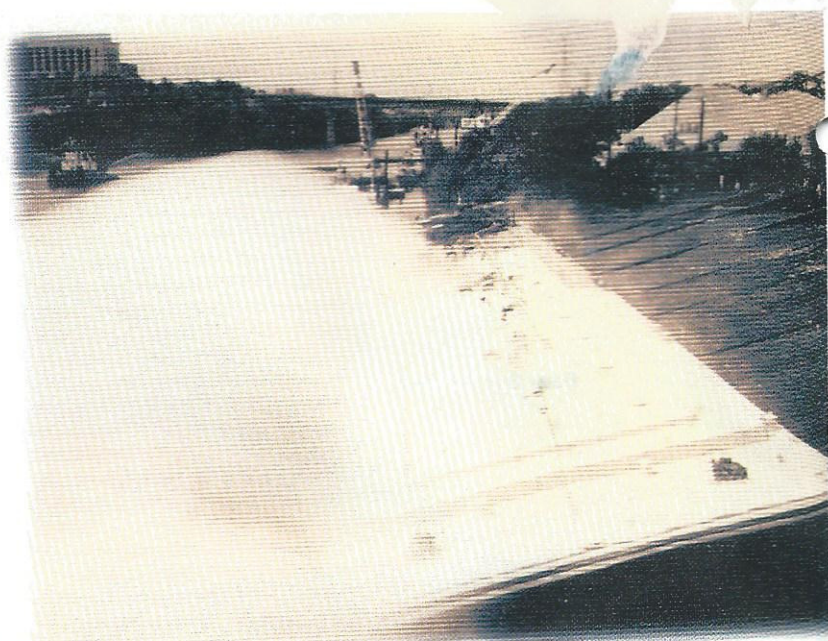
Barge STAR 2001, side launching into Cumberland River
